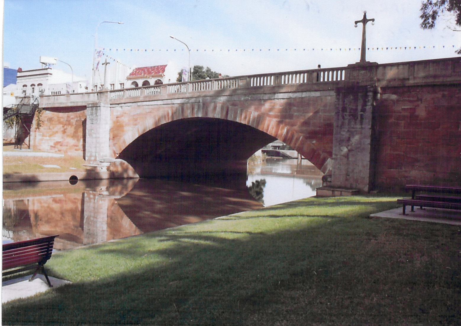
LENNOX BRIDGE, PARRAMATTA: STONE ARCH, 1839
