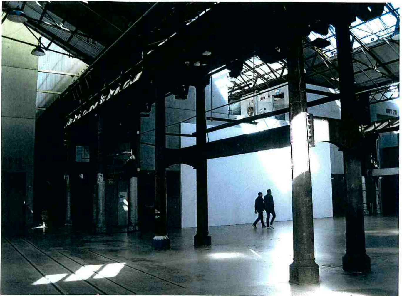
THE CARRIAGEWORKS, REDFERN, SYDNEY: CAST IRON COLUMNS, 1887
