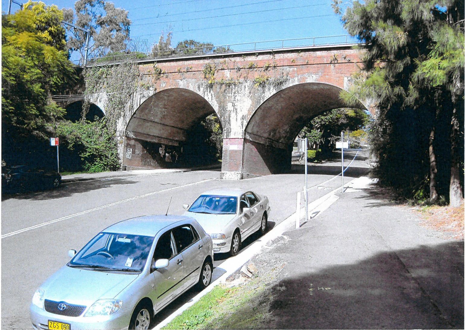
WOLLSTONECRAFT RAILWAY BRIDGE, SYDNEY: BRICK ARCHES, 1893
