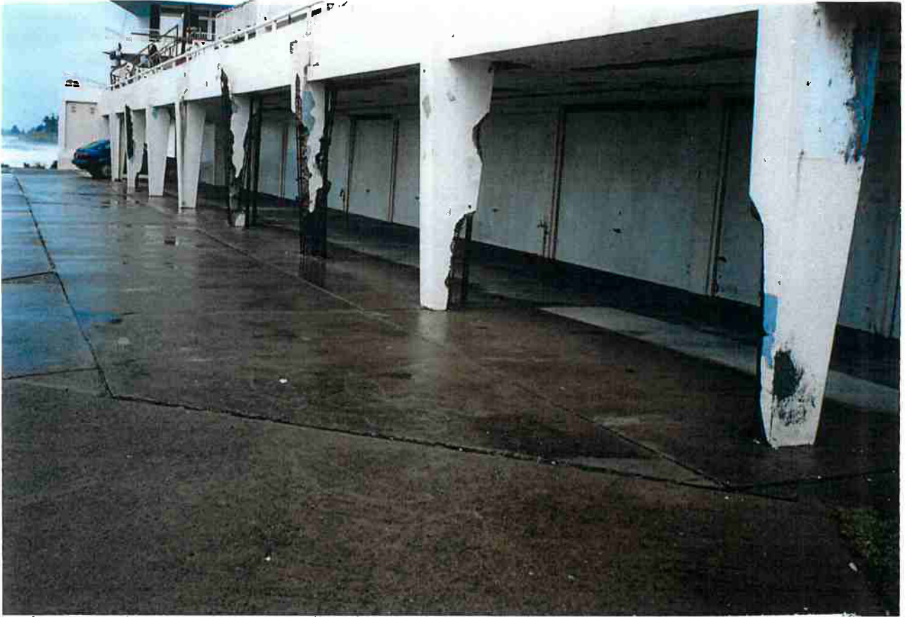
COLLARROY BEACH APARTMENTS, SYDNEY: REPAIR OF CONCRETE
