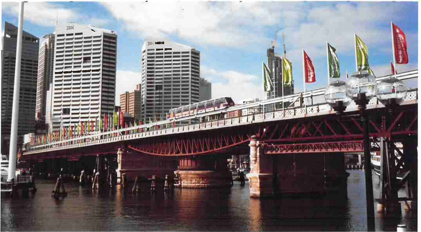
PYRMONT BRIDGE, SYDNEY: STEEL SWING SPAN/TIMBER TRUSS APPROACH SPANS, 1902
