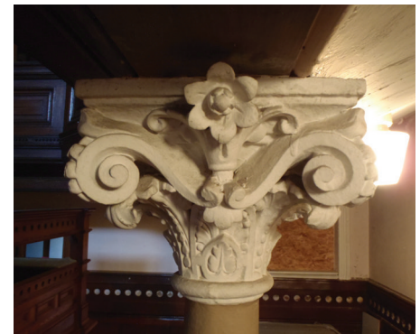
Figure 2 Cast iron column, complete with cast Corinthian capital
