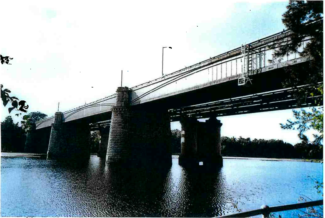
VICTORIA BRIDGE, PENRITH, NSW: WROUGHT IRON BOX GIRDERS, 1867
