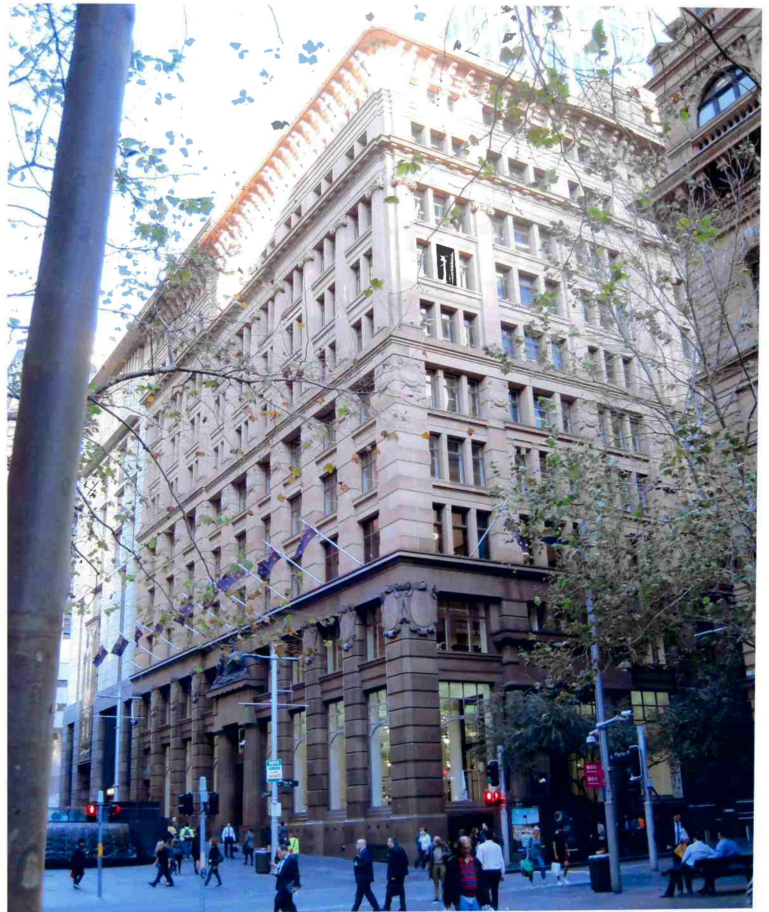
COMMONWEALTH BANK, SYDNEY: STEEL FRAME, 1916.
