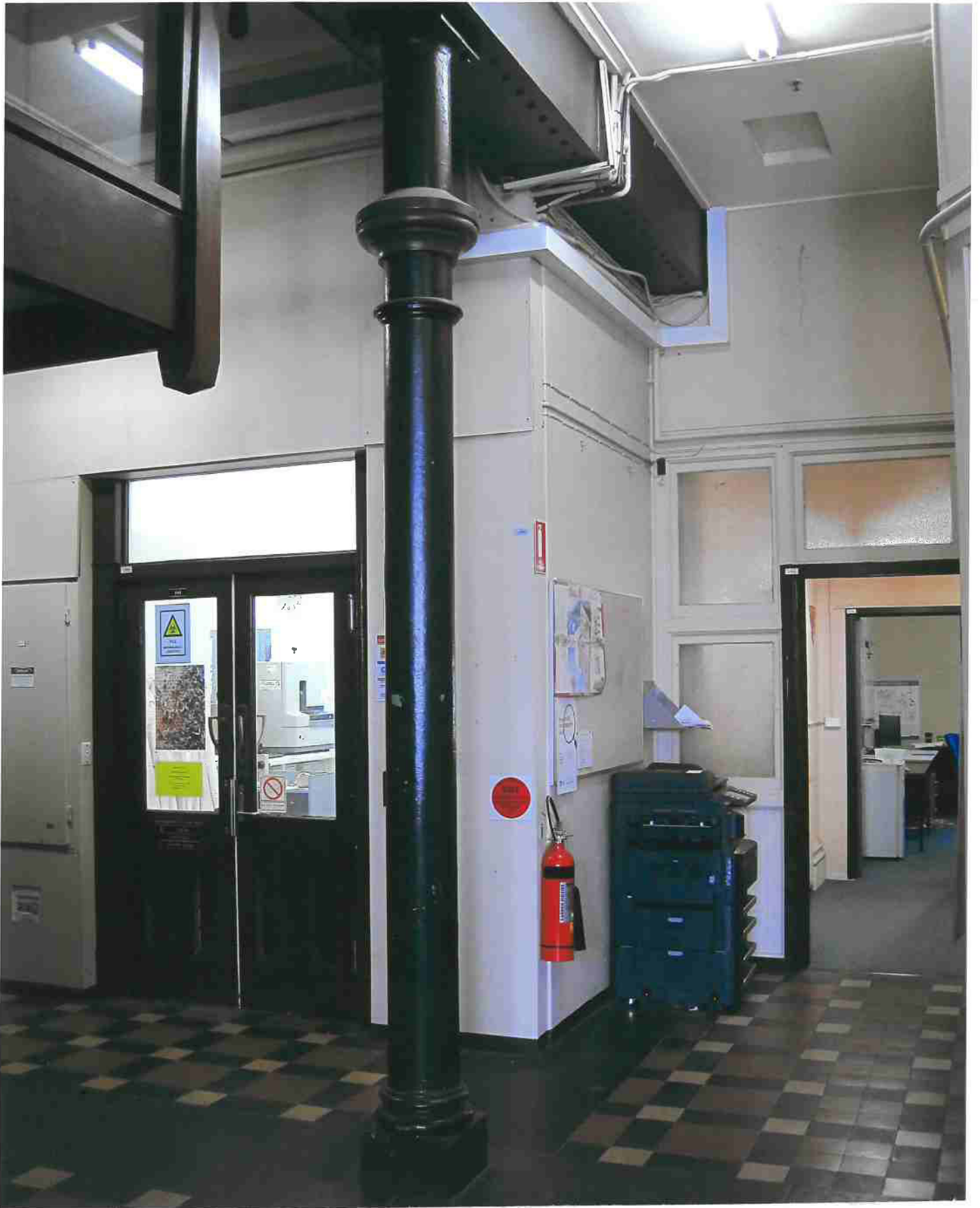
MACLEAY MUSEUM, UNIVERSITY OF SYDNEY: CAST IRON COLUMNS, 1887
