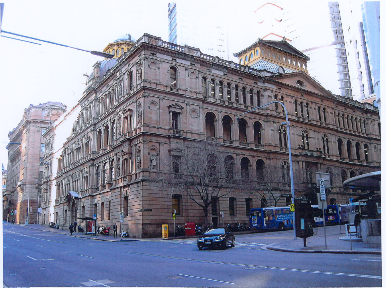
DEPARTMENT OF LANDS BUILDING, SYDNEY: SANDSTONE, 1876+
