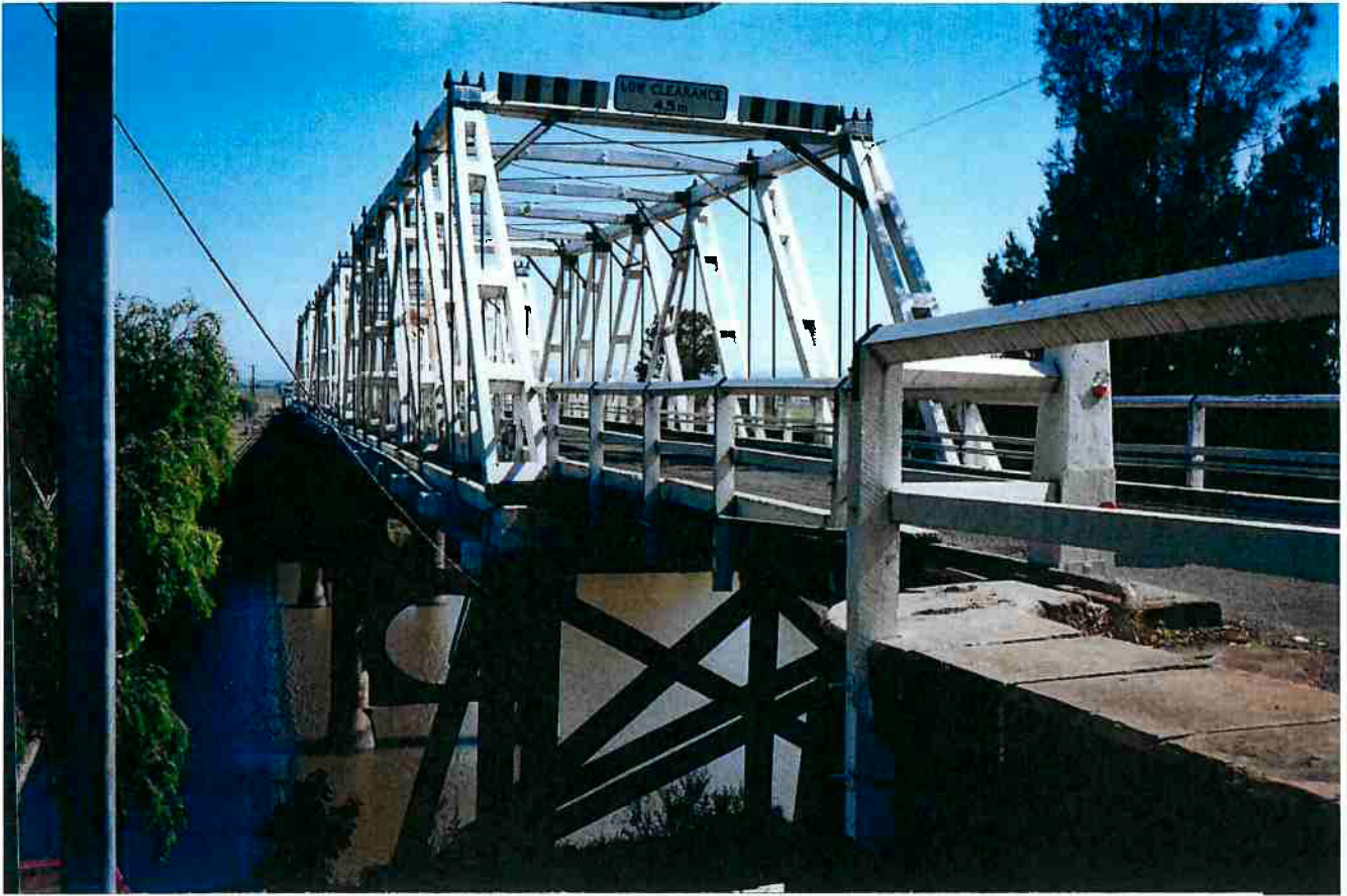
MORPETH BRIDGE, NEW SOUTH WALES: TIMBER ALLAN TRUSSES. 1898
