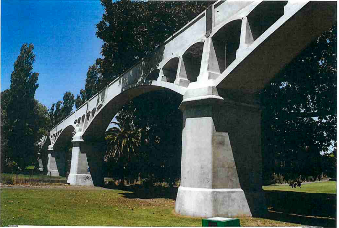
ANNANDALE SEWER AQUEDUCTS: REINFORCED CONCRETE ARCHES, 1896
