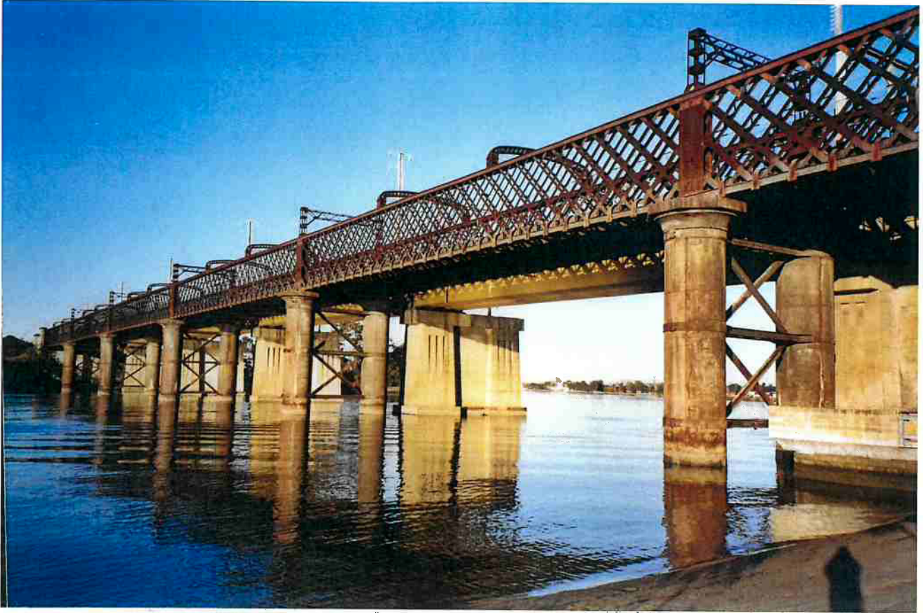
MEADOWBANK RAILWAY BRIDGE, NSW: WROUGHT IRON LATTICE SPANS 1886
